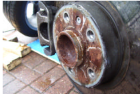
Above: Typical corrosion to hub flange face
